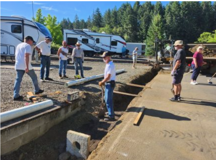
PCM at work on the Alder Way front lot drainage project.
