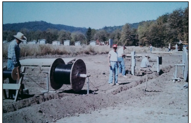
Prepping the land! Laying the lines.
